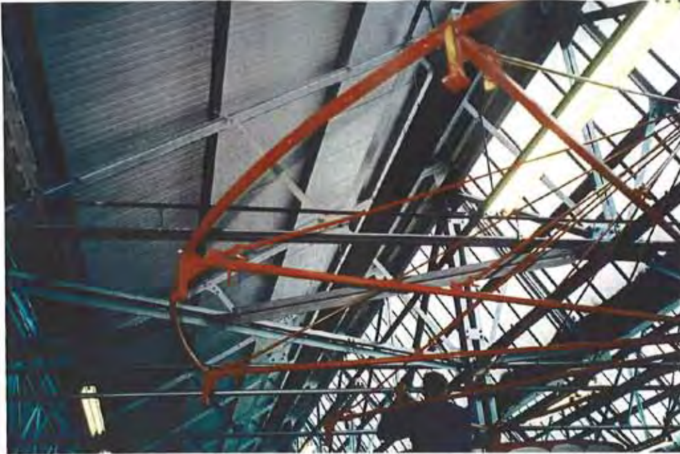
HOOK SUSPENSION RODS ON TO HORIZONTAL ROOF BARS. BOLT ON OUTER RING SECTIONS.
